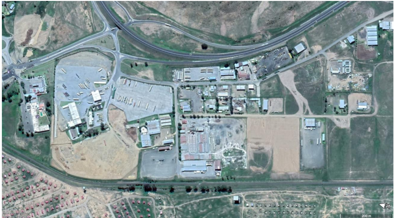
Figure 11: Highway Junction complex, Harindustria, Harrismith
